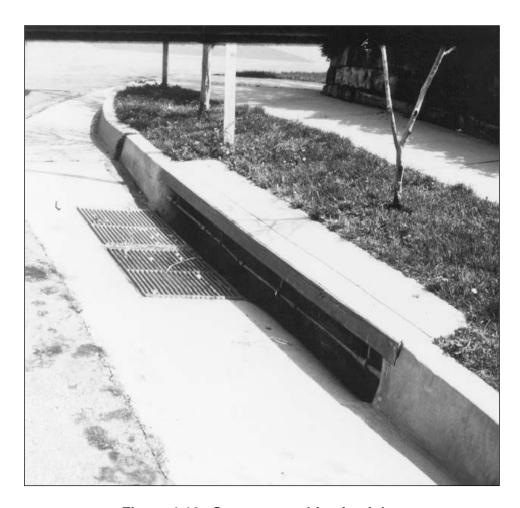
Figure 4-16. Sweeper combination inlet.
